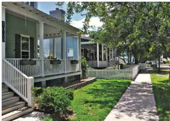
Prior to 1995, 10th Street in Port Royal, SC, was wide and treeless, and the lots were mainly empty. The town swapped some of the right-of-way for an alley in the back, creating a walkable, tree-lined street that made it attractive to build houses with porches facing the people-friendly thoroughfare.
