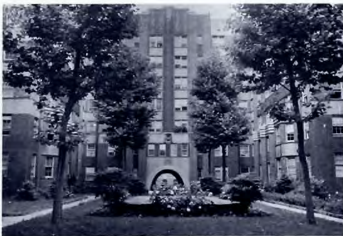
Fig. 55. Amalgamated Dwellings . Springsteen & Goldhammer, 1930. Courtyard view looking north.
