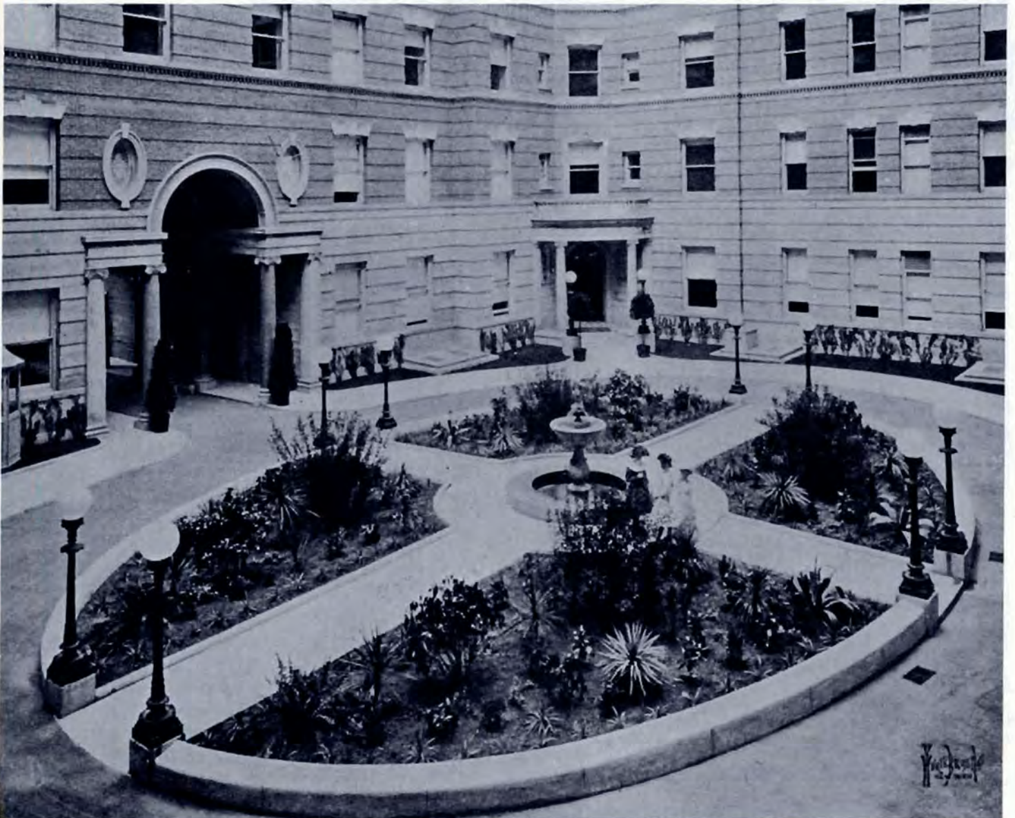
Fig. 28. Graham Court. Clinton & Russell. 1901. View of courtyard.
