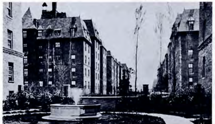
Fig. 45. The Towers . Andrew J. Thomas. 1924. View of garden.
