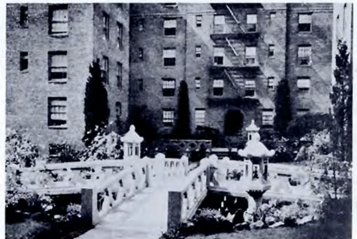
Fig. 52. Thomas Gardens. Andrew J. Thomas. 1927. View of courtyard from Grand Concourse. Fig. 54. Courtyard detail.
