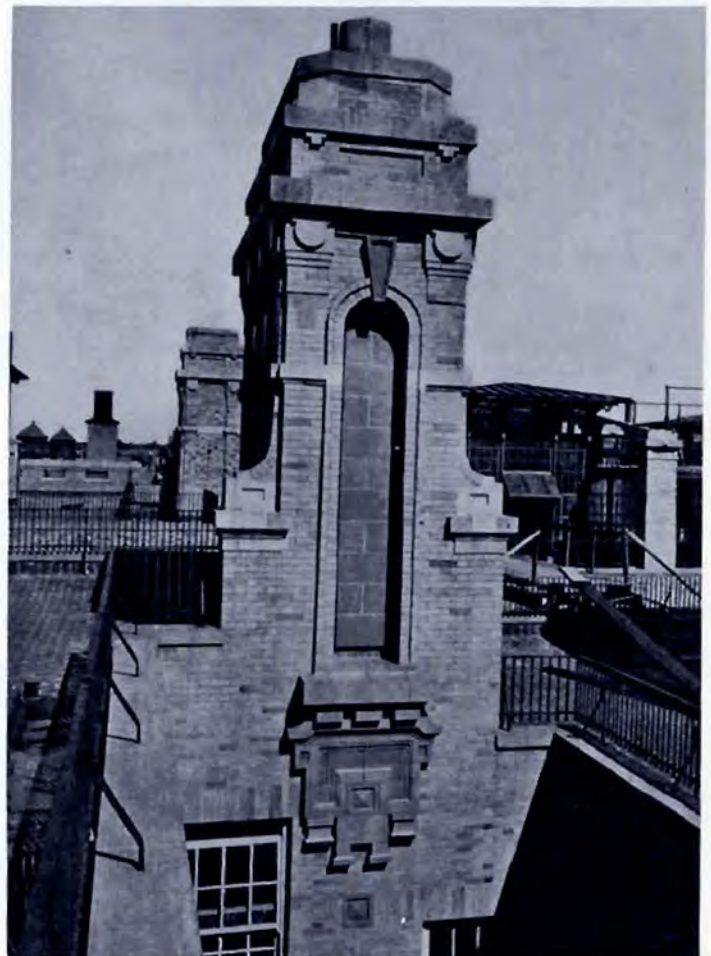
Fig. 18. East River Houses. Henry Atterbury Smith. 1908–1909. Chimney detail.
